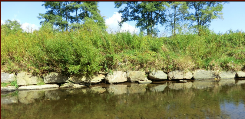
An example of a once-eroding streambank that has been repaired.
