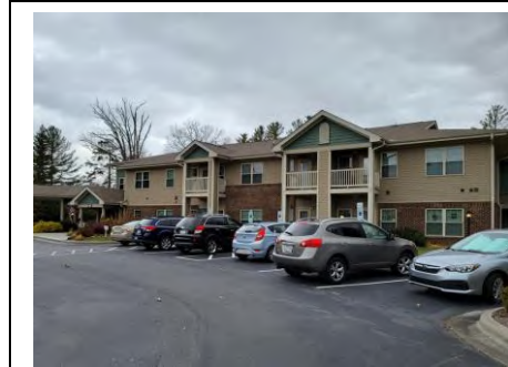
Linville Cove Apartments Newest (2013) Tax Credit Project (Fully Occupied, Senior 55+)
