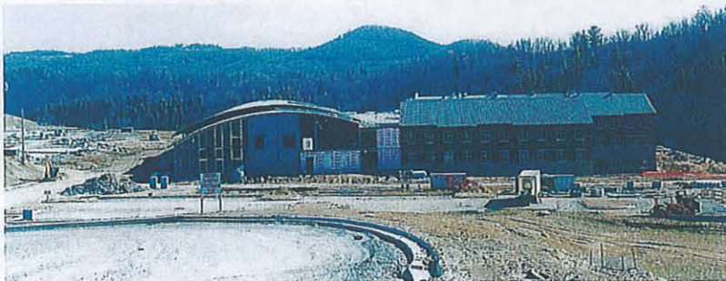
Watauga 1 High School under construction, March 2009
