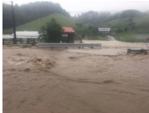
May 18, 2018 – one of several bridges over the Watauga River is over-topped impeding access residents and emergency personnel.
